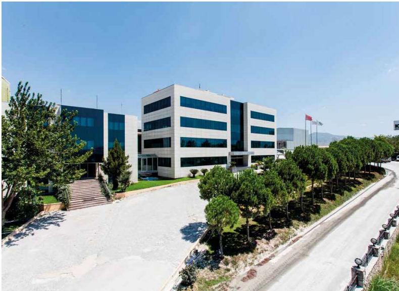
Fig. 1 Kaltun Mining Headquarters in Aydin/TR
