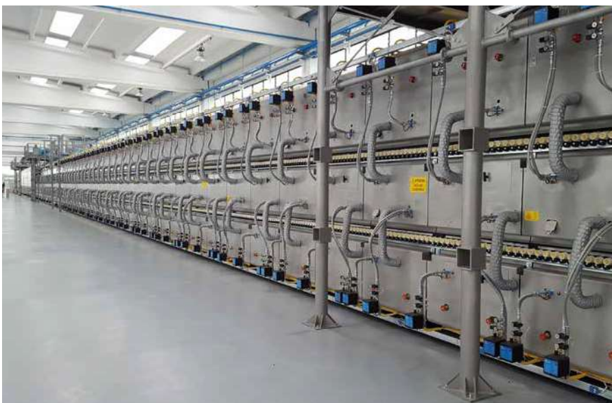
Fig. The new WFR kiln for firing large-format tiles
