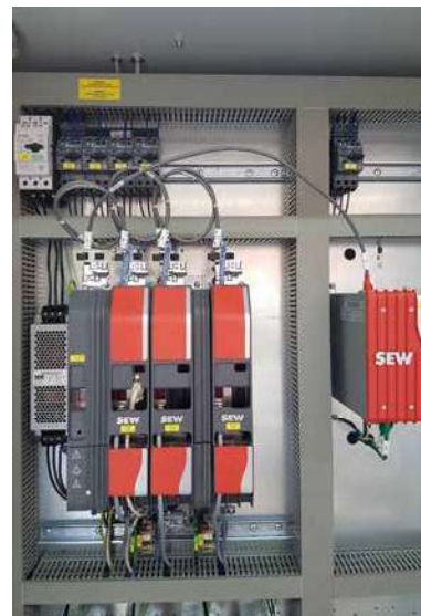
Fig. 1 The new SEW converter of the Movi-C generation (Source: KELLER)
