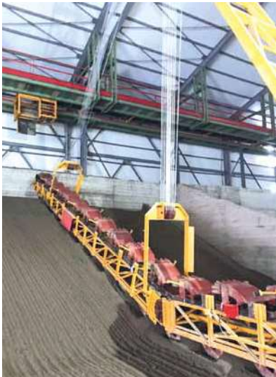
Fig. 3 Automatic silos excavator
